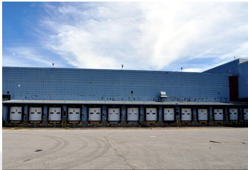
Space B: 14-bay loading dock
